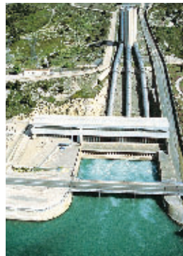
Hydroelectric power plant of Saint-Chamas, Marseille
